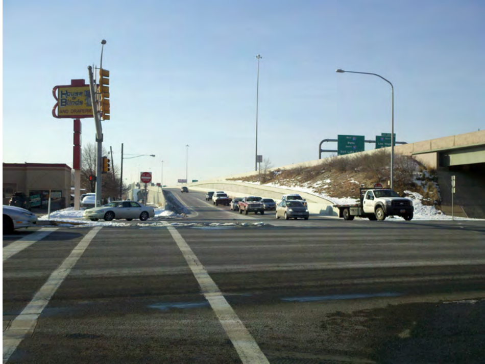
Figure 3. Typical view of the project area. Interchange of I-80 and State Street. View to the west.
