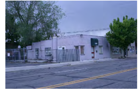
2386 S MAIN Eligible/Contributing
