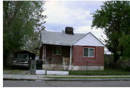
48 W 2400 SOUTH Inelig./Non-contributing
