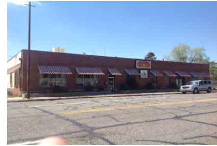
2470 S MAIN Eligible/Contributing
