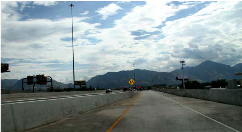
Eastbound Weave Area on I-80
