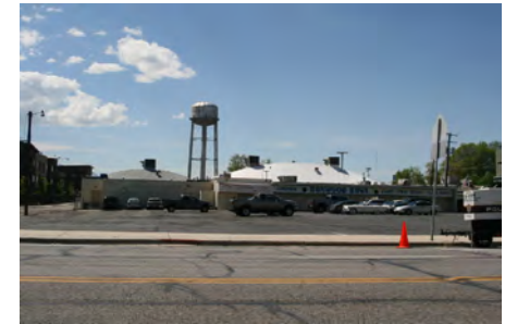
2500 S MAIN Eligible/Contributing
