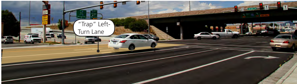
State Street at the I-80 Interchange Looking Northbound
