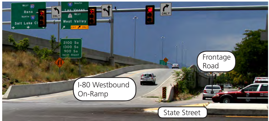
I-80 Westbound On-Ramp and Frontage Road Looking West
