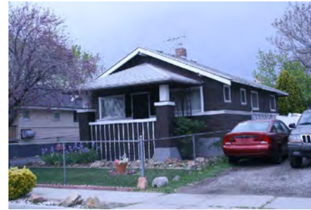
129 E WHITLOCK AVENUE Eligible/Contributing
