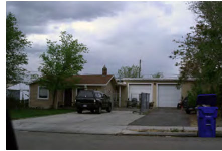
54 W 2400 SOUTH Inelig./Non-contributing
