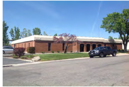
400 W LAWNDAL DRIVE Eligible/Contributing
