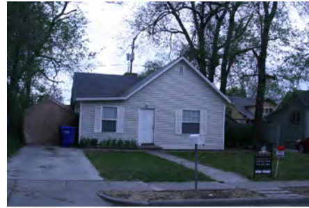
41 W ROBERT AVENUE Inelig./Non-contributing
