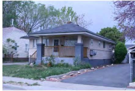
125 E WHITLOCK AVENUE Eligible/Contributing
