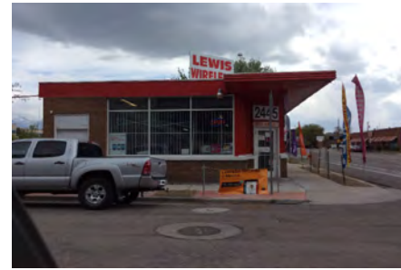
2445 S MAIN Eligible/Contributing
