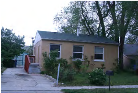
37 W ROBERT AVENUE Inelig./Non-contributing
